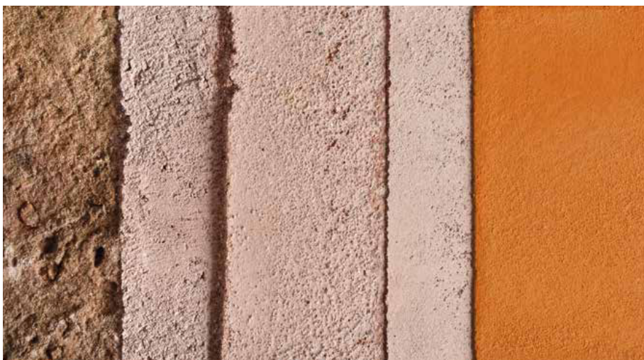
Facade stratigraphy composed of: stone structure, render in rialto malta grezza blended with cocchiopesto powder, layer of malta grezza blended with cocchiopesto , malta fine blended with cocchiopesto , rialto antiqua 1 finish.
